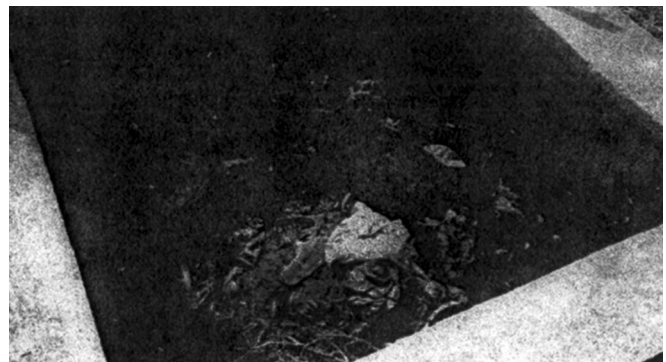
Fig. 13.5 Deep burial—a pit for disposal of organic (biodegradable) waste Source: Govt. of Karnataka. Karnataka Health Systems Development Project Management of Hospital Waste 2001.
